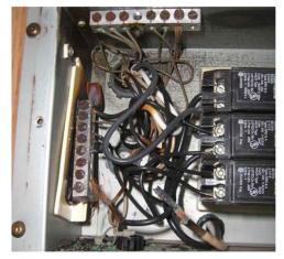
This damage was due to loose connections on the neutral bus bar, it got hot and melted the wires!
