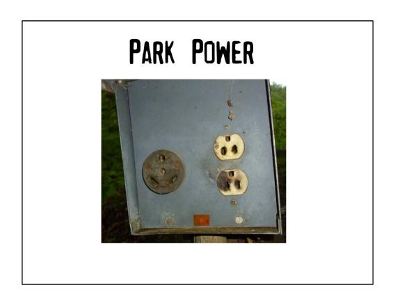
This is an example of a very old pedestal. Notice the burned receptacle and the lack of a disconnect or circuit breaker.
