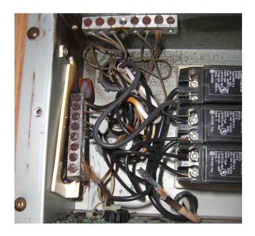
This RV panel damage was due to poor connections on the neutral bus bar, it got hot and melted the wires! The breaker did not trip!
