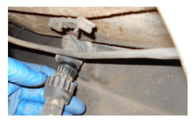
When you reassemble, attach a pull cord to the AC wires before you put the unit back on the ground to make easier to pull the wires back into the conduit.
