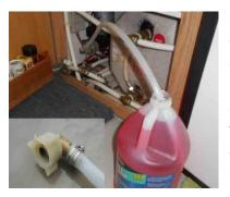
Unscrew the fitting which connects to the pump inlet and attach a hose with the other end inserted into a bottle of RV antifreeze. You can get the fitting and tubing at Home Depot or Lowes.
