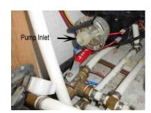
Turn on the pump. It will draw a small amount of antifreeze, but the pump should stop.
